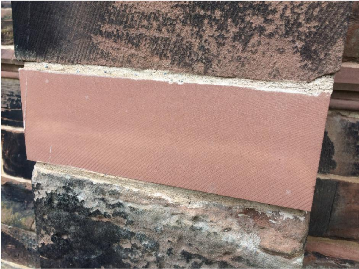
Fig.2: Circular saw marks still visible of new masonry units.
